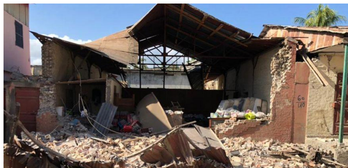
A 7.2-magnitude earthquake that struck Haiti this month killed thousands and caused widespread damage. A partially collapsed building in the city of Jérémie is pictured. // Photo: USAID.
