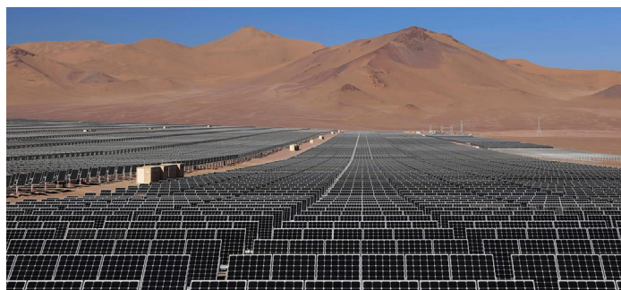
The Cauchari Solar Park in Argentina, the largest one in South America, was constructed with financing from the Export-Import Bank of China. // File Photo: Argentine Government.
