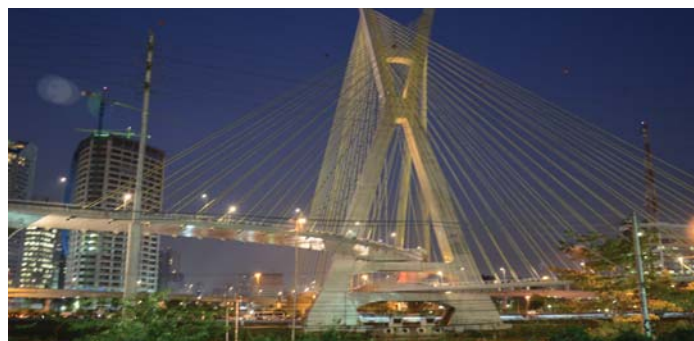
The Octávio Frias de Oliveira bridge, which opened in 2008, has become one of São Paulo's most recognized landmarks // File Photo: Rodrigo Soldon via Creative Commons license.
