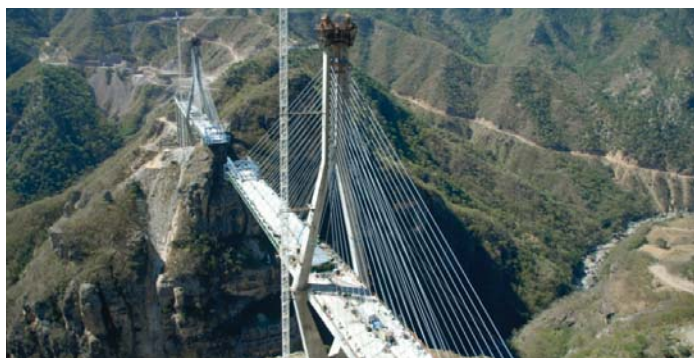
Leaders of multinational lenders have expressed concerns that the Trump administration may cut funding to the lenders that would normally go to project finance in Latin America. Mexico's Baluarte Bridge, before its completion, is pictured above. // File Photo: Grupo Tradeco.
